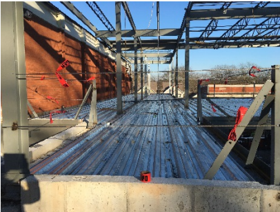
Elevated Decking, Structural Steel Erection, & Exterior Framing
