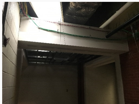
Hard Ceilings Installed
