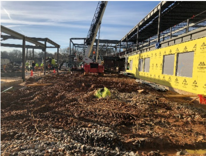
Structural Steel Erection, Stairs, & Exterior Framing/Sheathing
