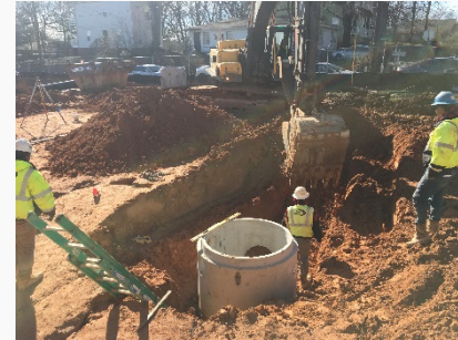
Installation of Yard Inlet Behind Retaining Wall
