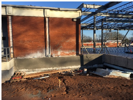
Backfilled and Waterproofed Retaining Wall
