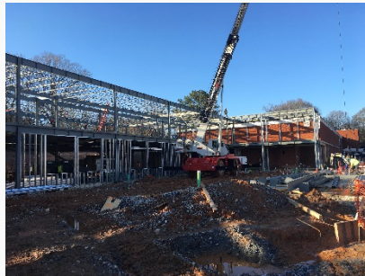
Elevated Decking, Structural Steel Erection, & Exterior Framing
